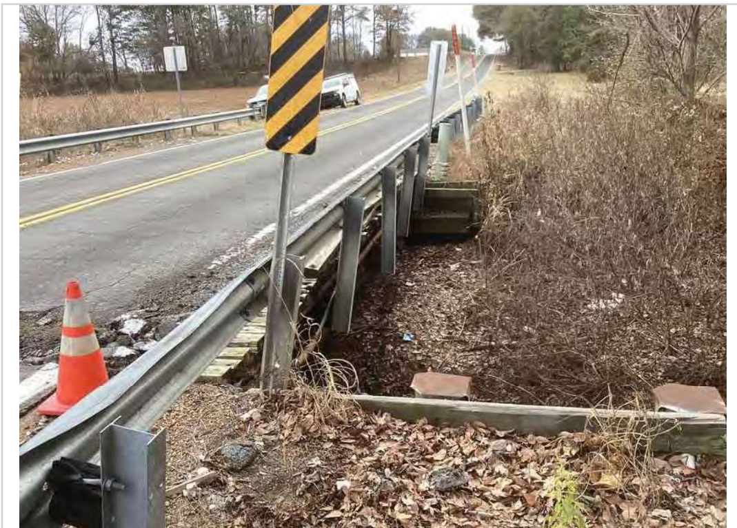
Left side rails not connected span 1
