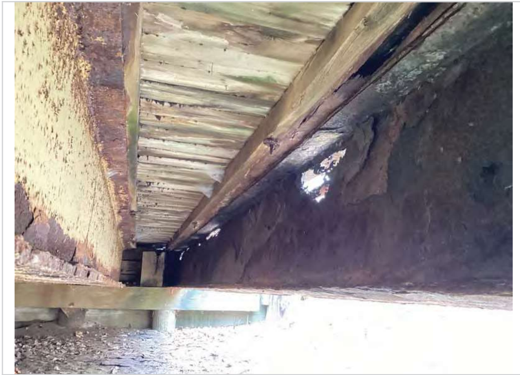
Steel I beam "A" span 1 (Holes in web) & bottom flange
