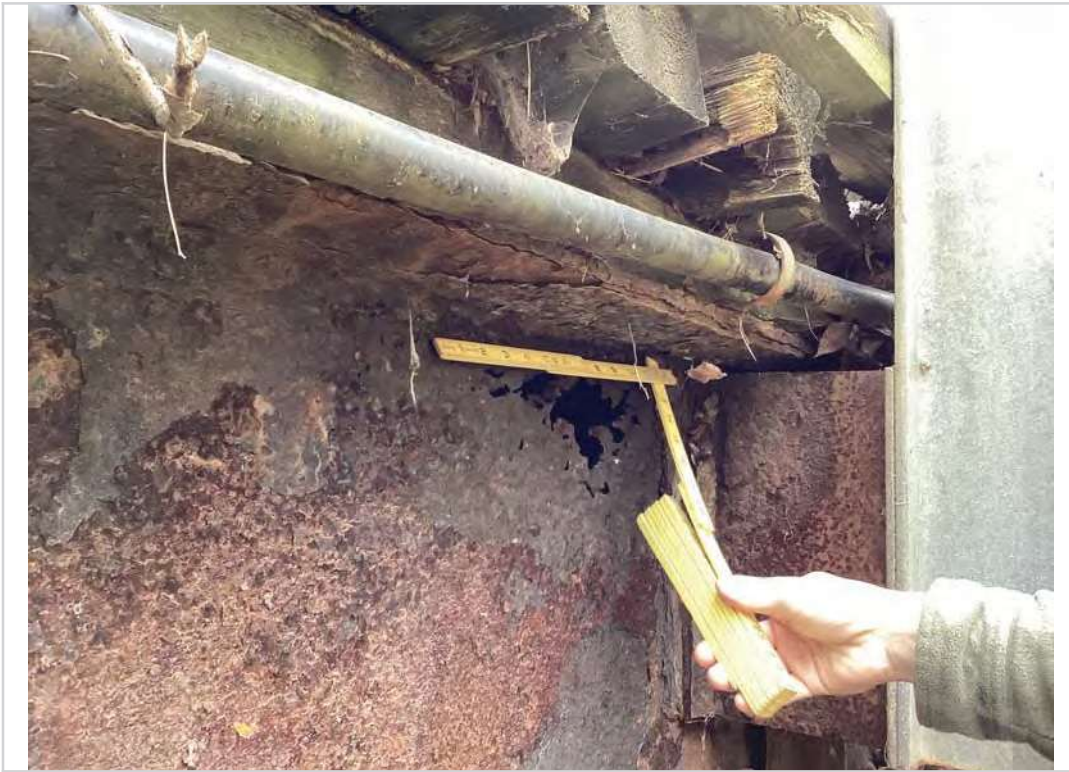
Steel I beam "A" span 1 (hole in web) beginning of span
