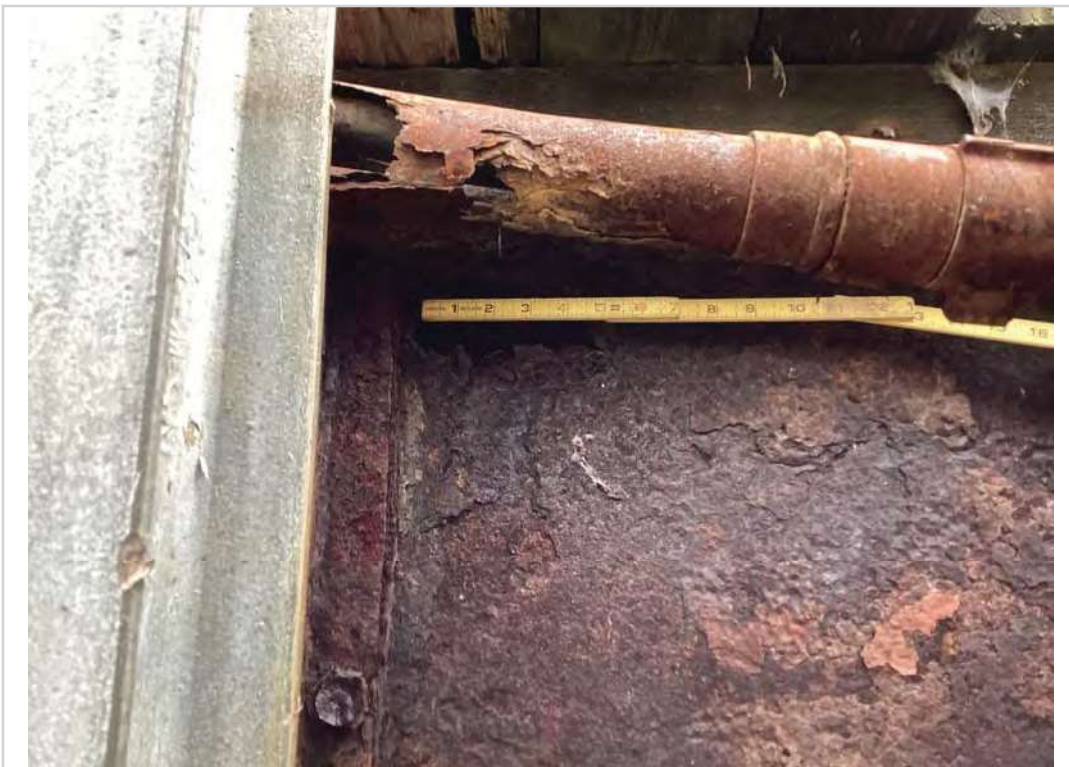
Steel I beam "A" span 1 (hole in web)
