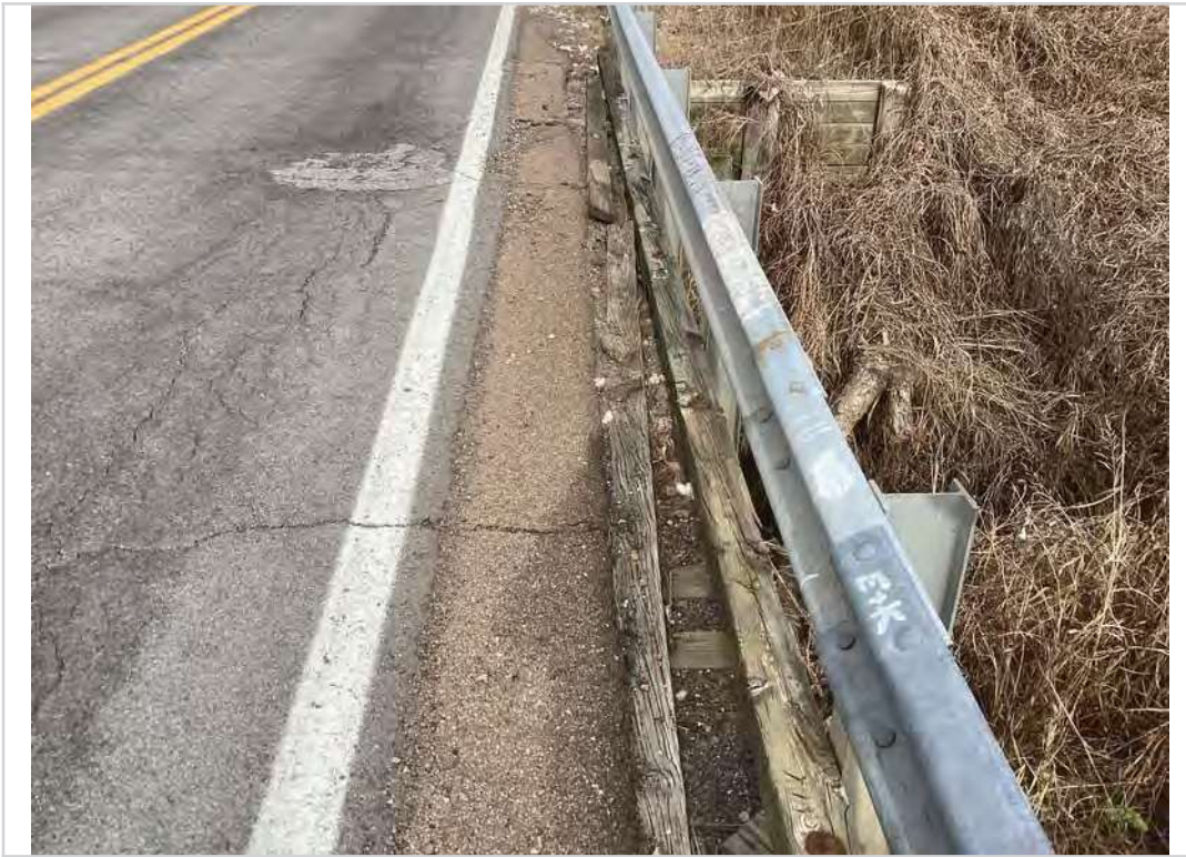
Rtside wheel guard broken and missing span 1
