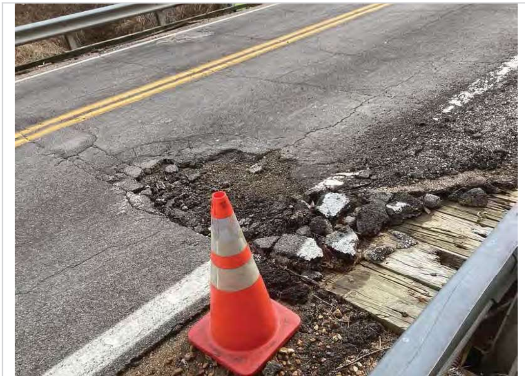
Approach 2 asphalt spalling
