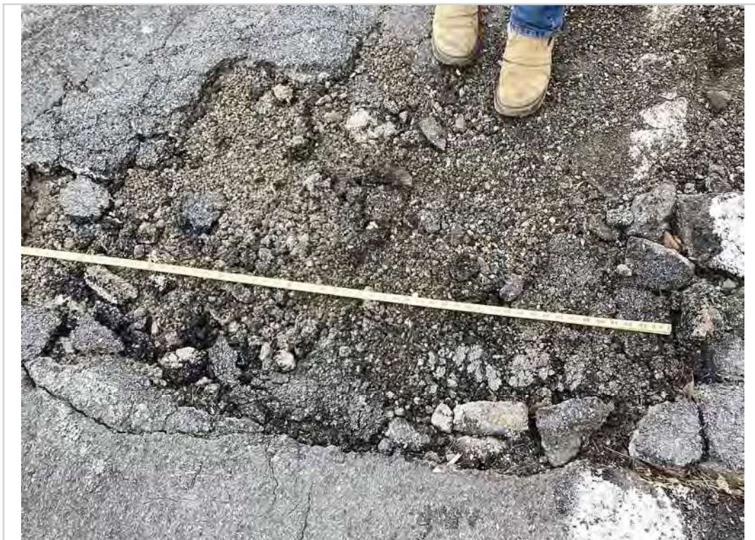
Span 1 spalling area on approach 2 side left side
