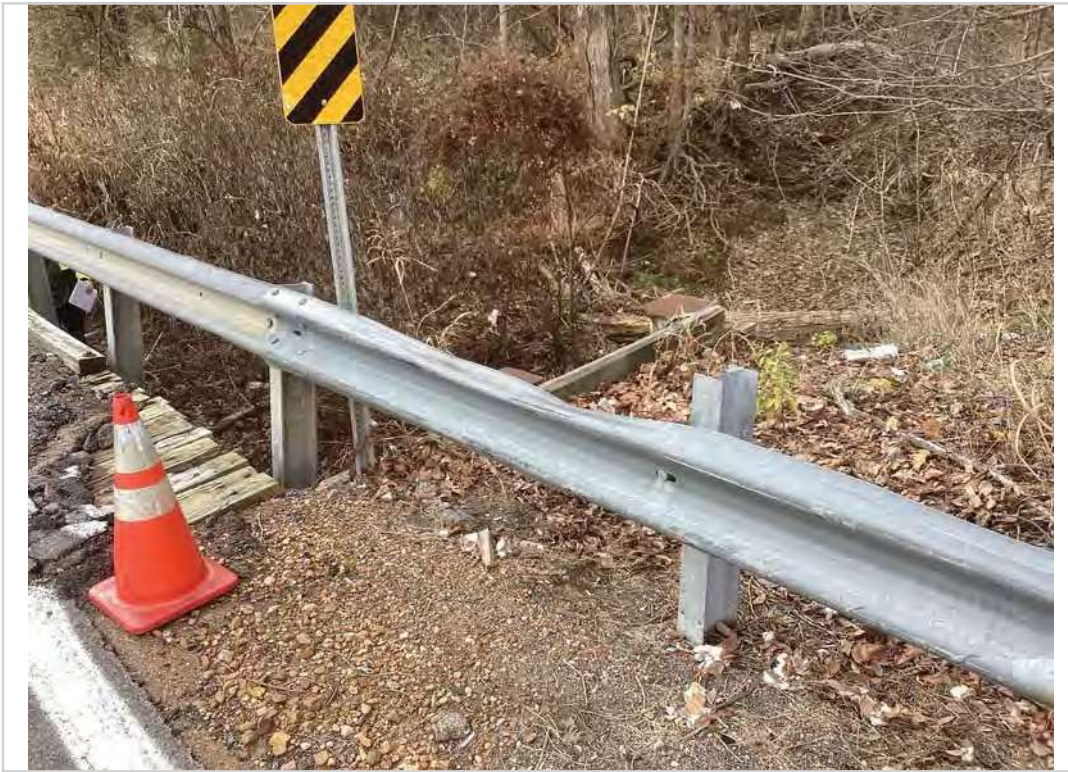
Left side approach 2 bridge rail collision damage
