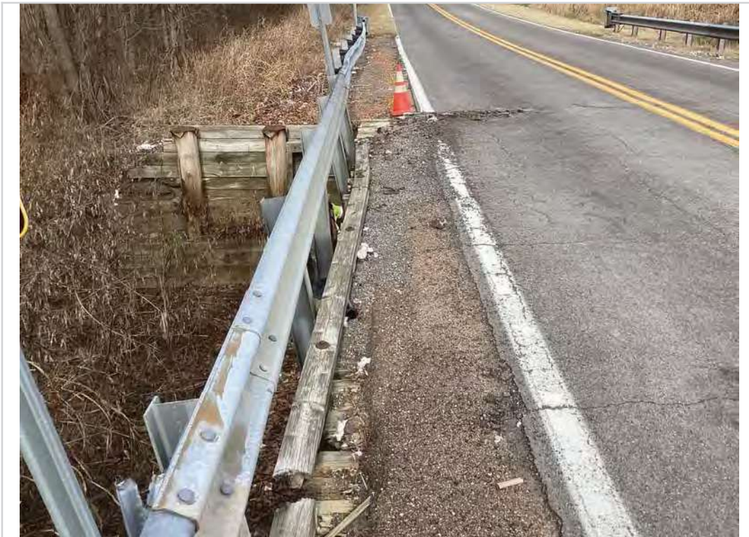
Left side span 1 wheel guard broken and missing
