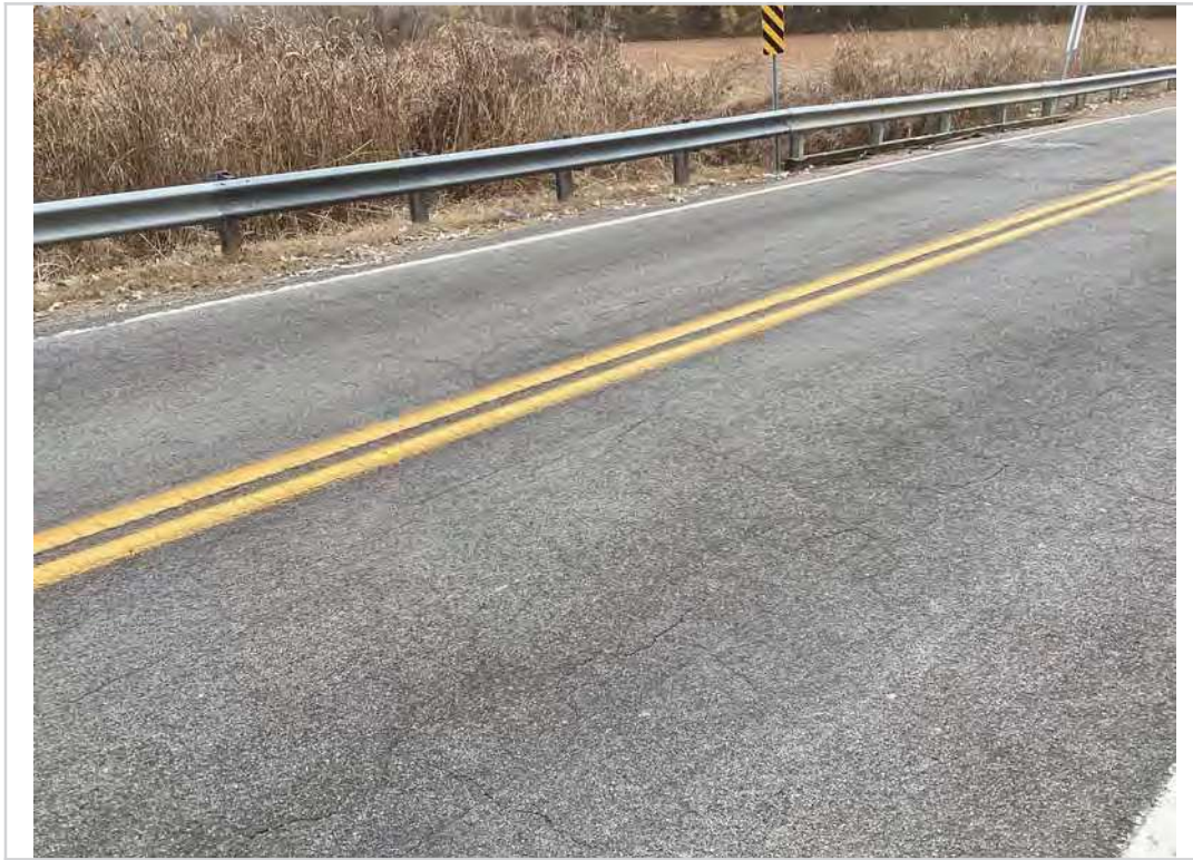
Span 1 top deck up to 1/4" cracks
